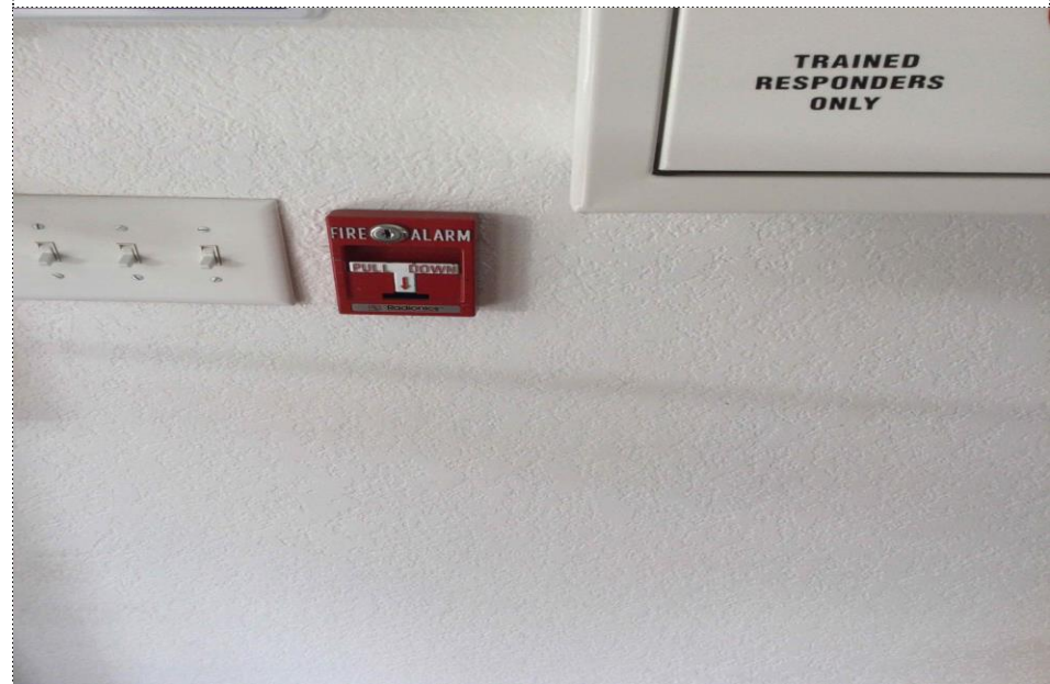
Typical Existing Pull Station
